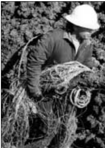
This major telephone cable would not have been cut if the contractor had done the proper checking beforehand.
