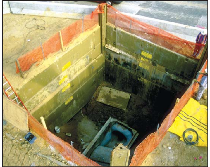
A slide rail shoring system protects workers in a 24-foot deep trench.
