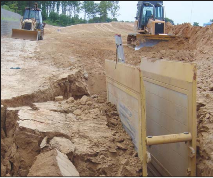
When this trench collapsed in East Arkansas, a shield protected workers.
