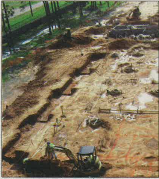
Site work progresses on footers, slabs and underground utilities.
