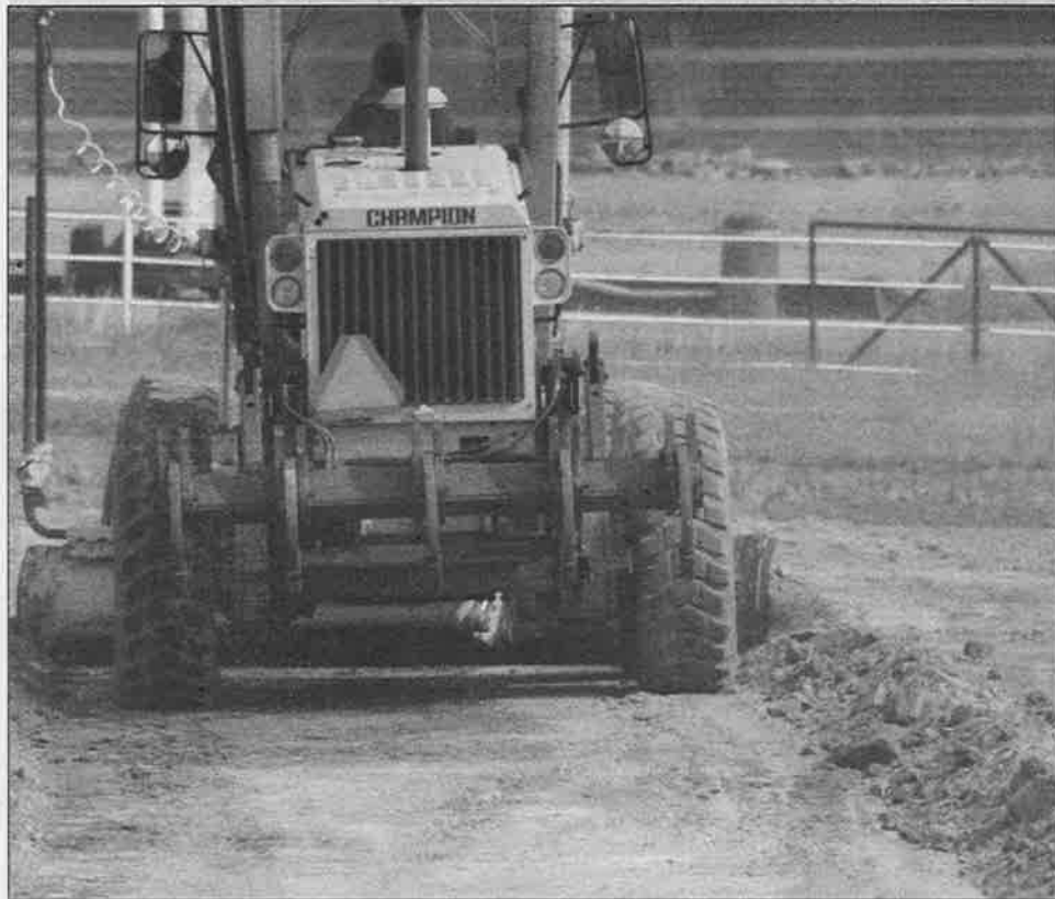
The motorgrader leaves behind a smooth grade.
