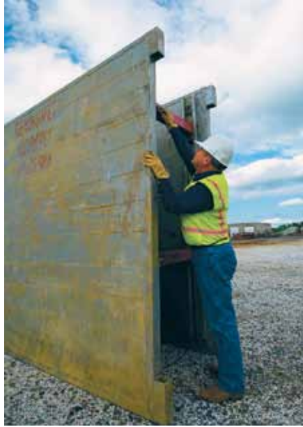
A “competent person,” as specified by OSHA, inspects an aluminum trench prior to use. Photo courtesy of TrenchSafety & Supply Inc.
